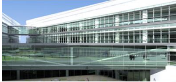
Sancaktepe Engineering Center (2015)
