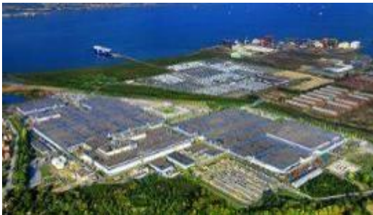
Kocaeli Plants: Gölcük Plant: Transit (2001), Custom (2012)
