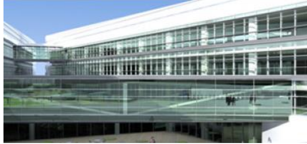
Sancaktepe Engineering Center (2015)
