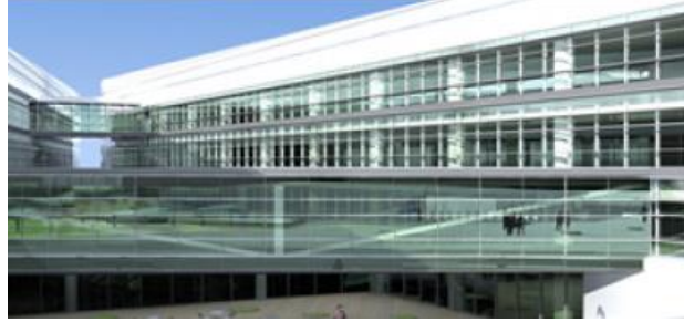
Sancaktepe Engineering Center (2015)
