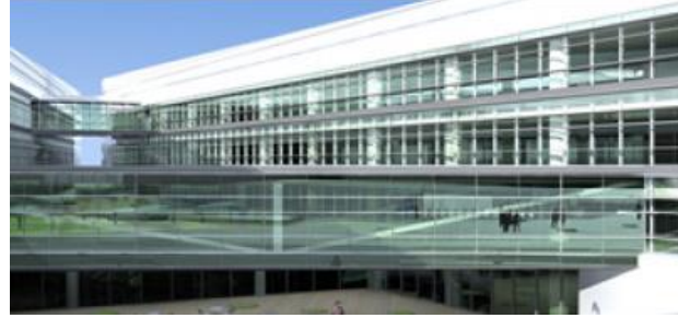
Sancaktepe Engineering Center (2015)
